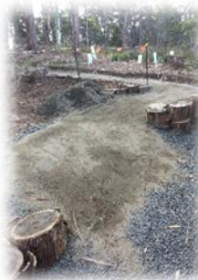
Crusher dust on path and drain cleaned out on western side of range.
