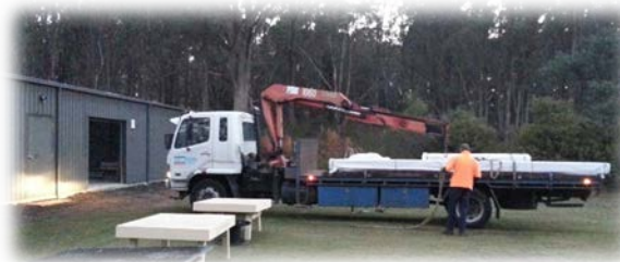
7am delivery for the Safety Wall build.29/3/2018
