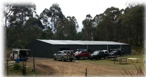
Electricians and plumber hard at work. 2/3/2018
