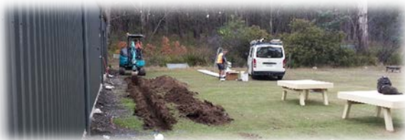
Plumber completing the drainage Fri 23/3/18
