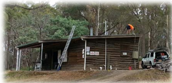
Security fitout under way. 2/3/2018
