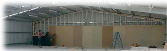
Then the sheeting
