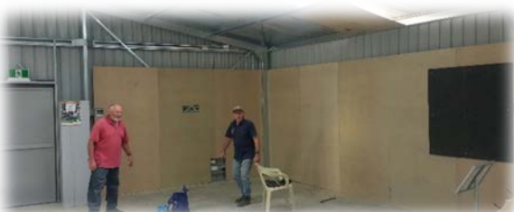
Brian and Barry fitting out the training area.
