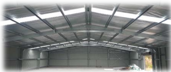
Still plenty of light now the roof is on.
