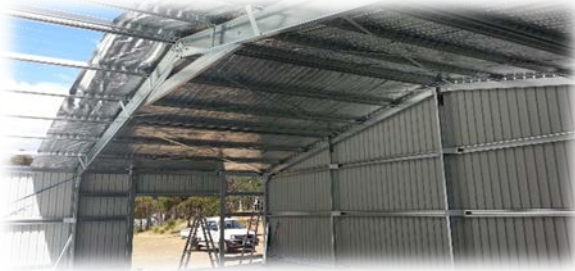
Sisalation going in on the roof.
