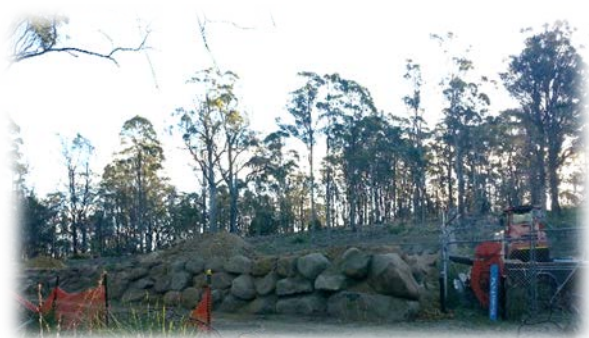
Preparation for the Rangers new shed, as seen from the road.
