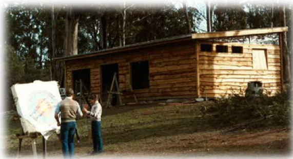
Construction of club house.
